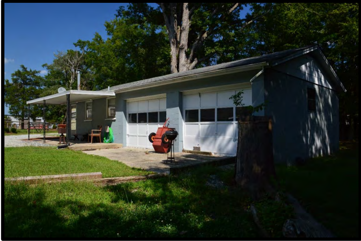
Figure 31: C.M. McLean House (GF8974), Secondary Dwelling, Looking Northeast.
