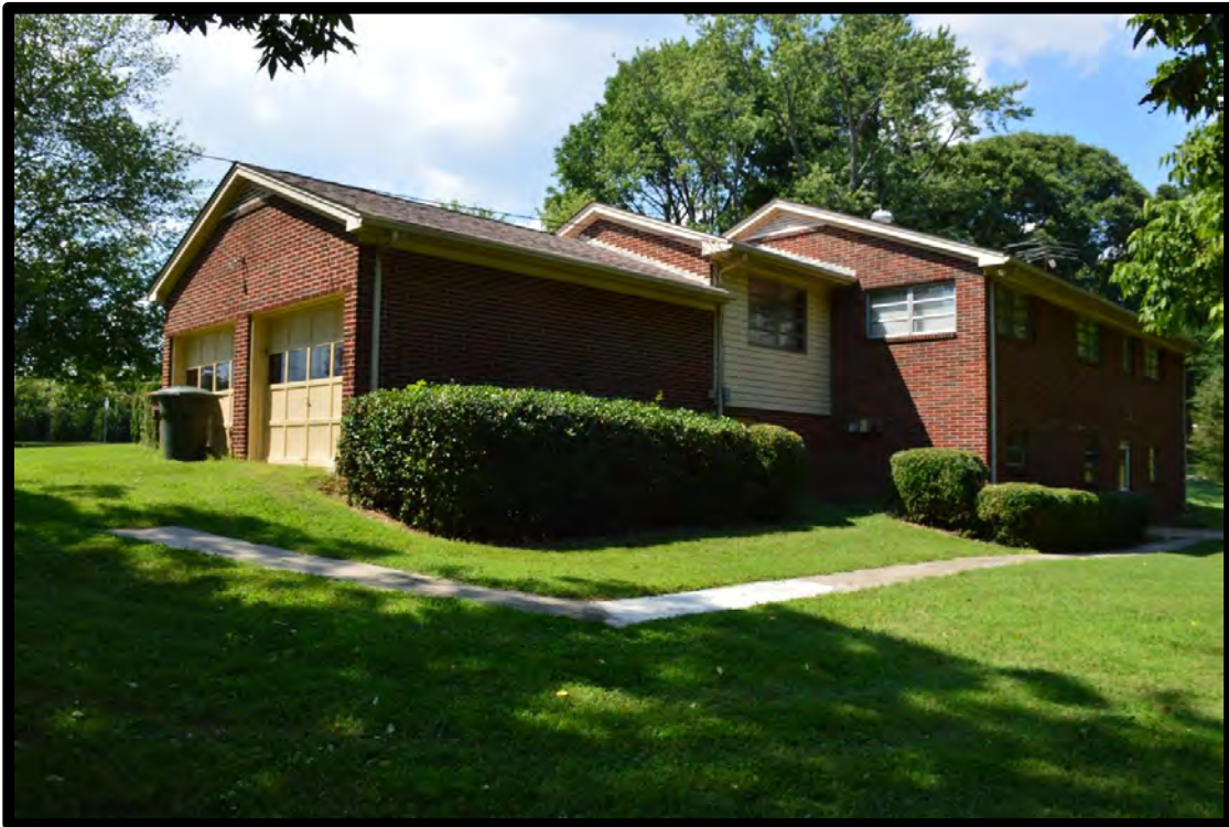
Figure 22: O'Ferrell House (GF8975), Looking Northwest.
