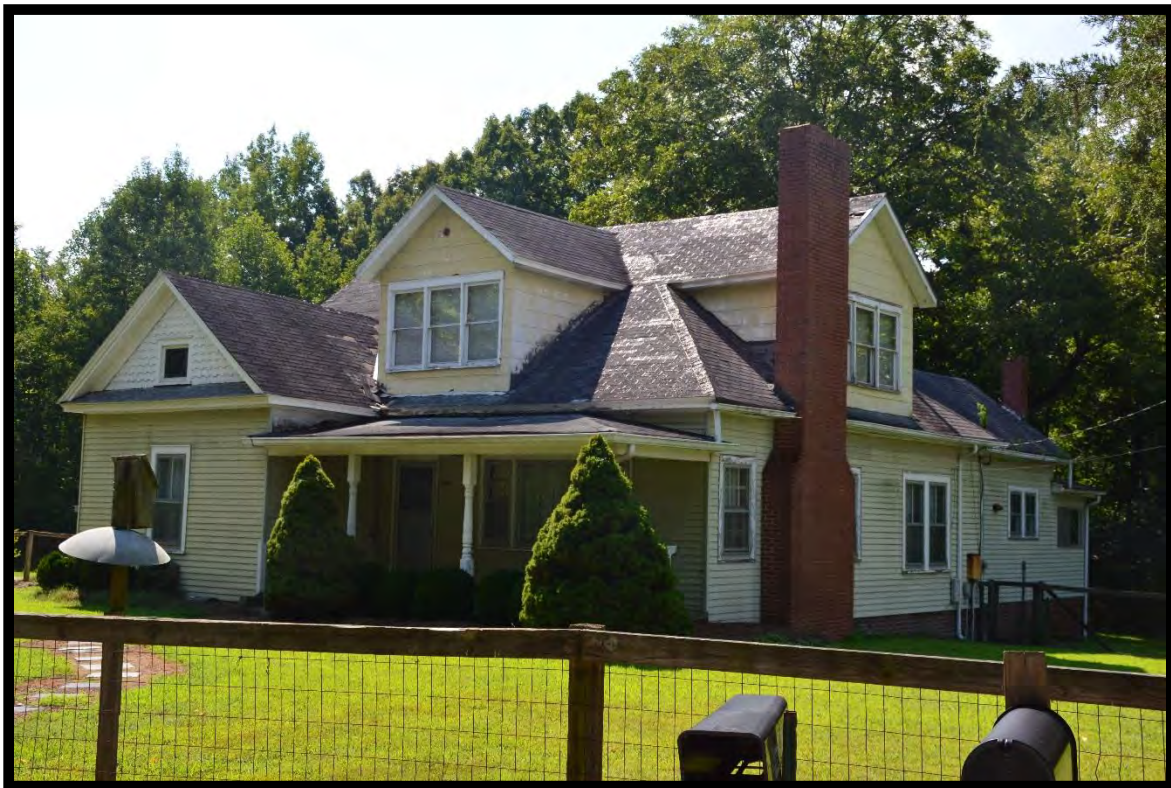
Figure 25: C.M. McLean House, 126 Maxfield Road (GF8974), Looking Southwest.
