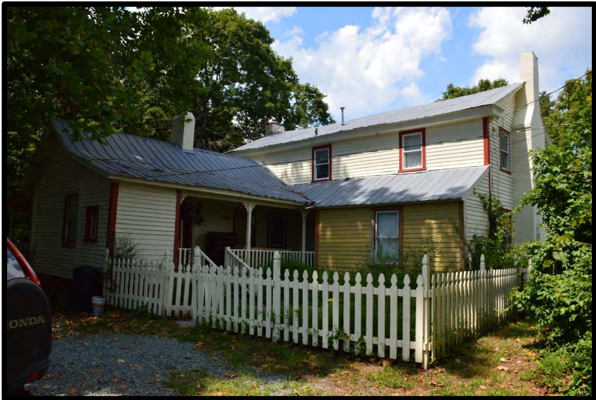
Figure 6: Buchanan House (GF6169), Looking Northwest.
