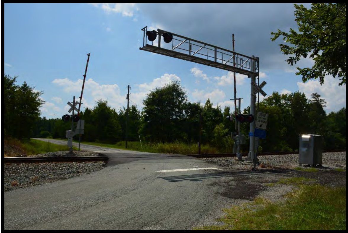
Figure 16: North Carolina Railroad (GF8976), Wagoner Bend Road, Looking Southwest.
