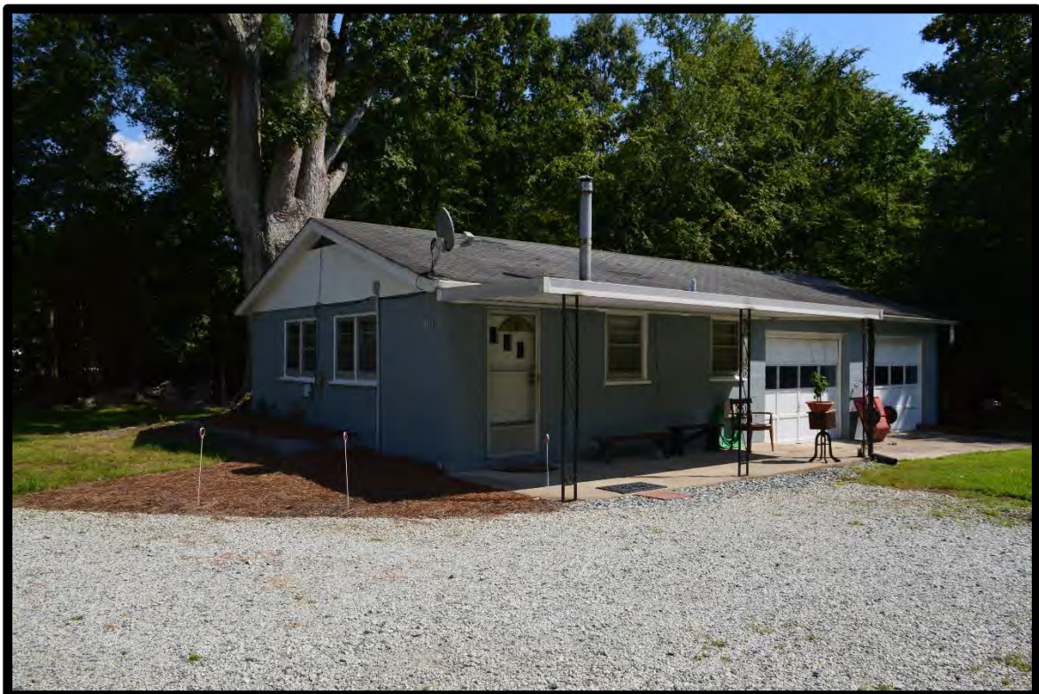
Figure 30: C.M. McLean House (GF8974), Secondary Dwelling, Looking Southeast.
