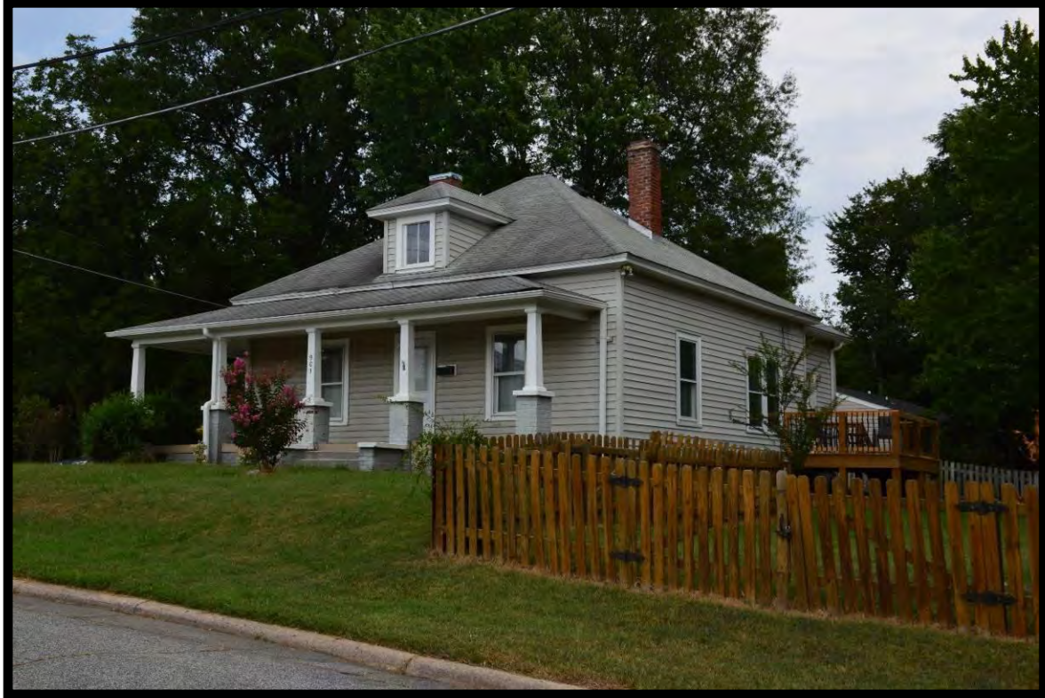
Figure 43: John R. Foy House, 901 McCormick Street, Greensborough, Looking Northeast.
