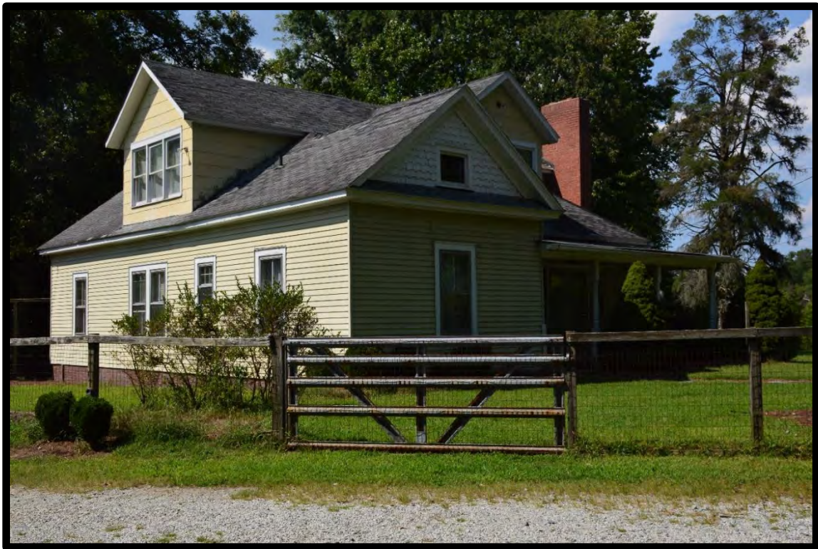
Figure 28: C.M. McLean House (GF8974), House, Looking Northwest.
