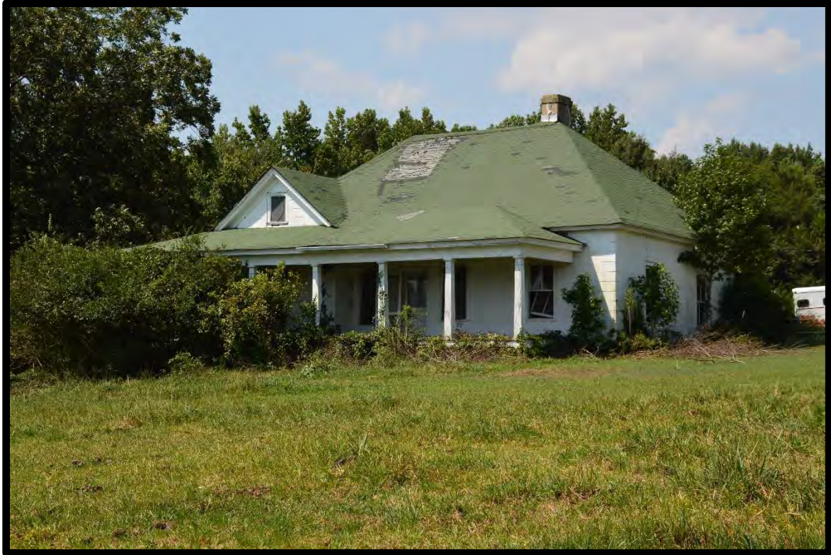
Figure 35: 3635 McConnell Road, ca. 1915 Queen Anne Cottage, Looking Northwest.
