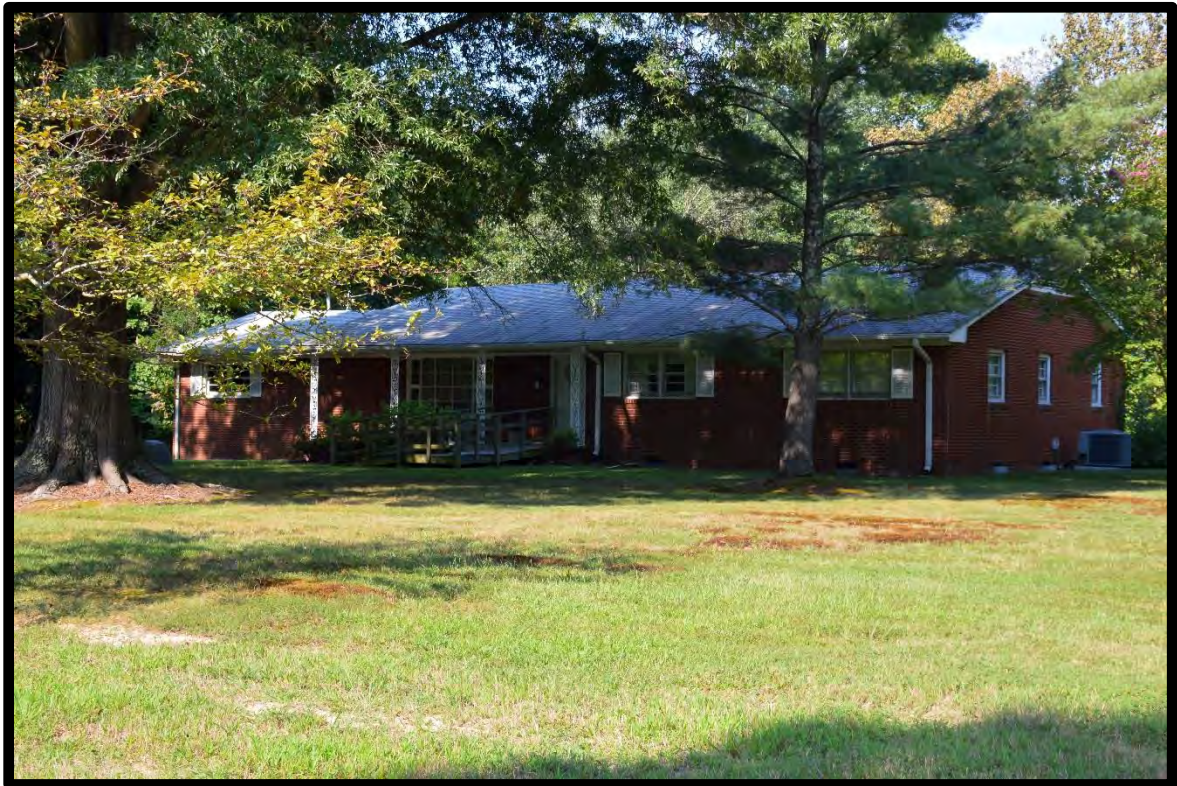
Figure 24: 1110 Mt. Hope Church Road, Looking Southwest.
