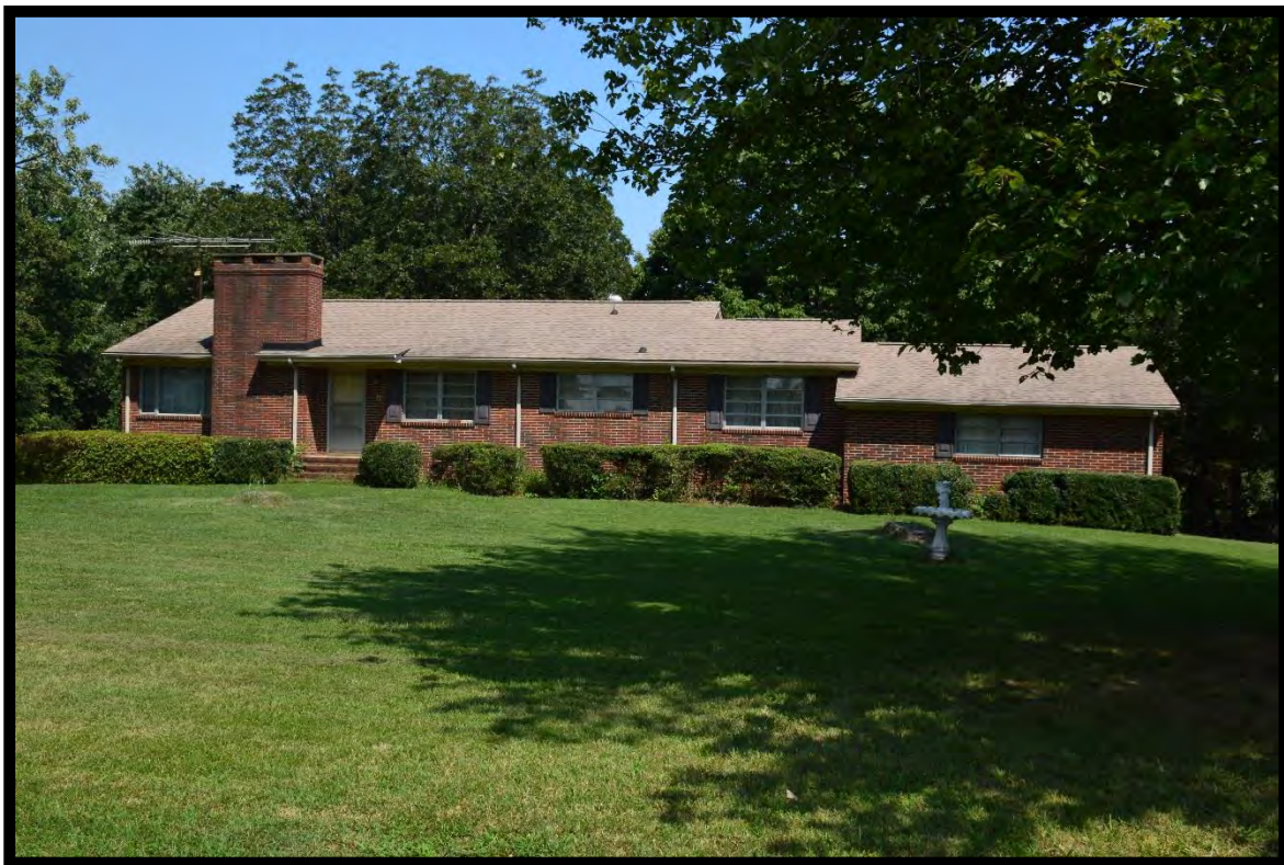
Figure 19: O’Ferrell House, 425 O’Ferrell Street (GF8975), Façade.
