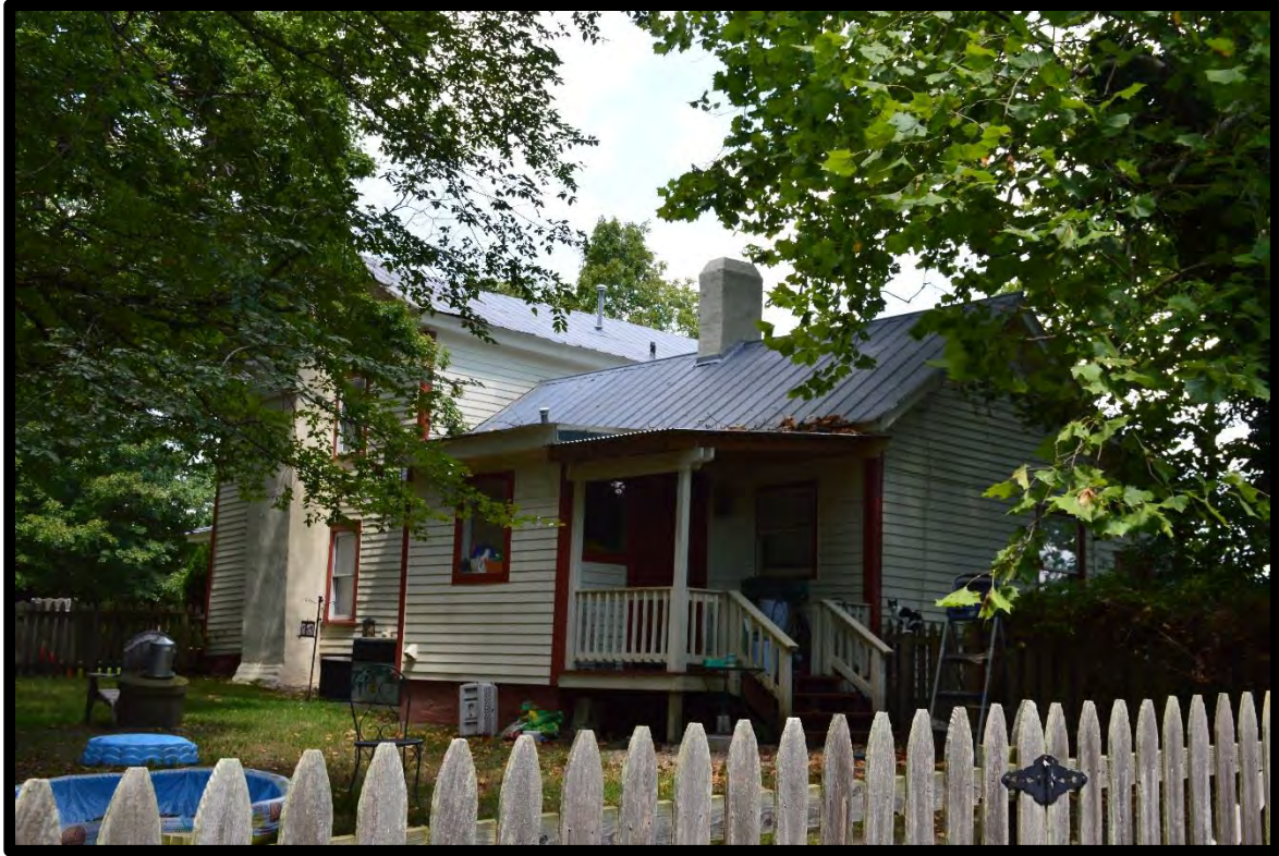
Figure 7: Buchanan House (GF6169), Looking Northeast.
